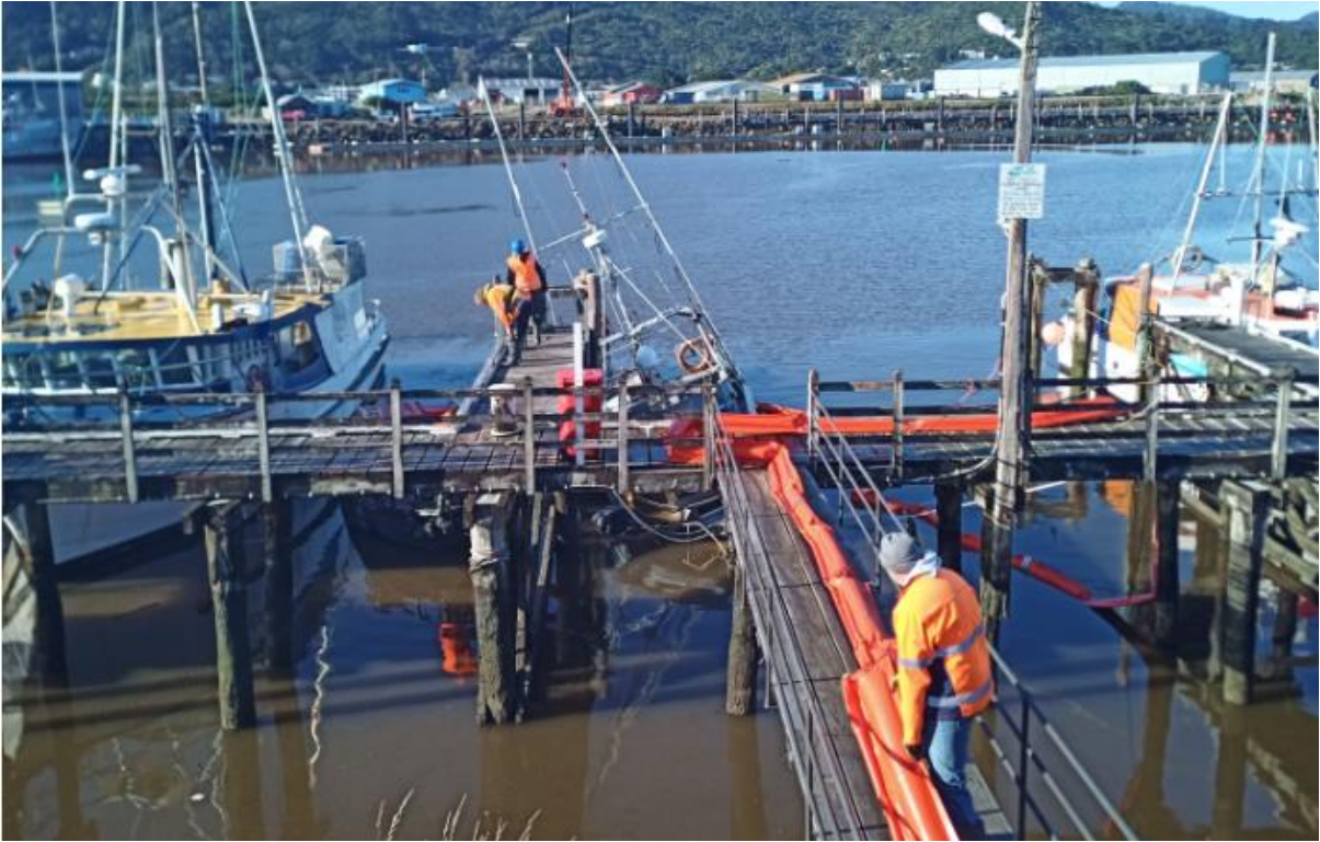
Figure 3: Rapid deployment boom being deployed:
